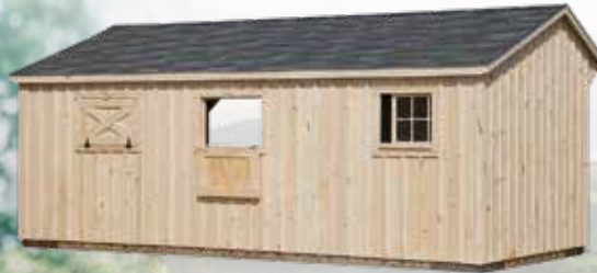
Run In Shed with Drop Vent
