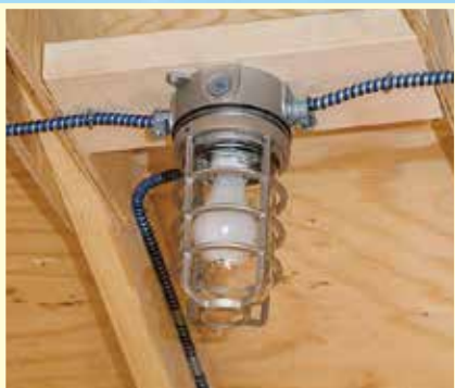
Vapor proof lights with die cast guard
