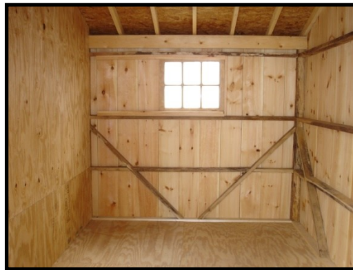
Interior view of tack room
