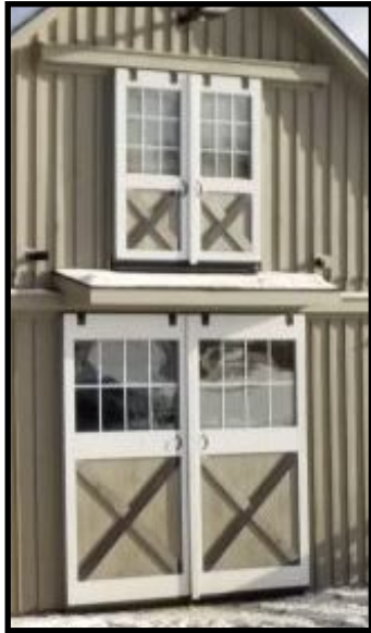
Double Sliding Doors Above Center Aisle
