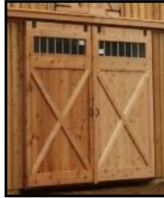
Transom Windows in Aisle Doors
