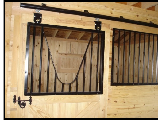
Sliding stall door w/ yoke in door
