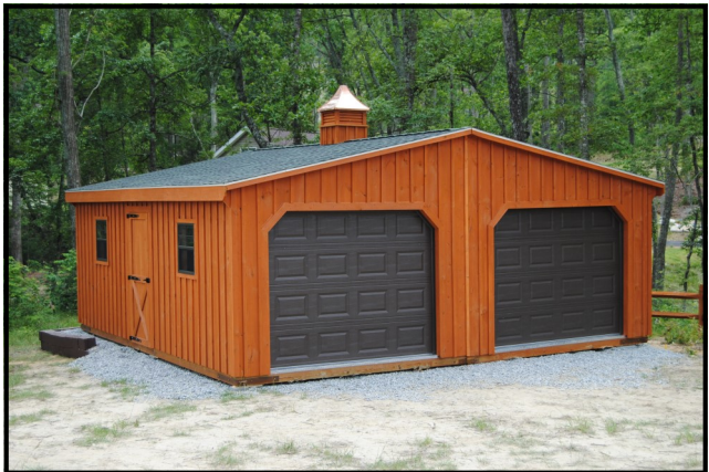
Completed garage in a few hours!
