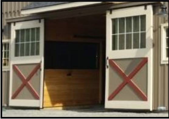
Tempered Glass In Aisle Doors
