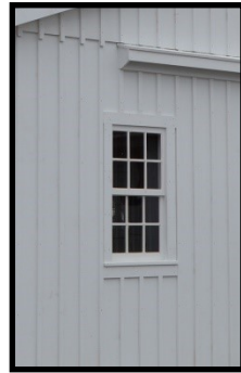
28"x48" Single-Hung Wood Sash Window
