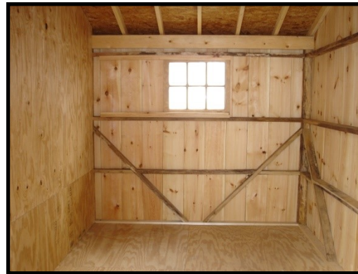
Interior view of tack room
