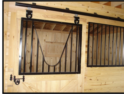
Sliding stall door w/ yoke in door
