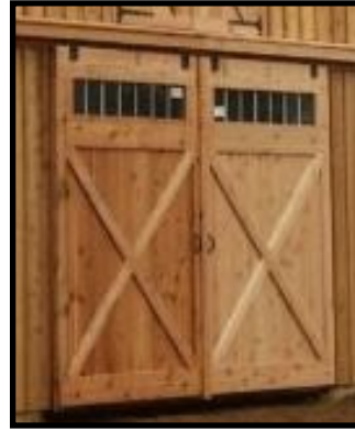
Transom Windows in Aisle Doors
