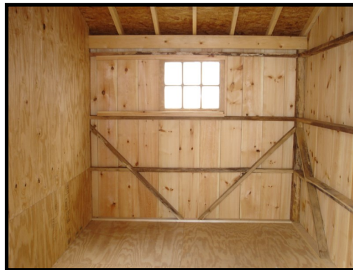
Interior view of tack room
