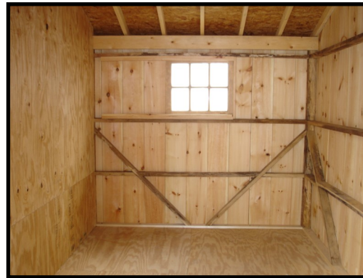
Interior view of tack room
