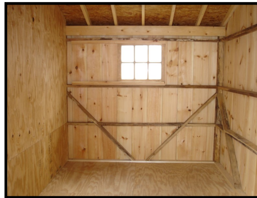
Interior view of tack room
