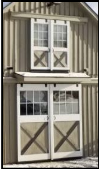
Double Sliding Doors Above Center Aisle
