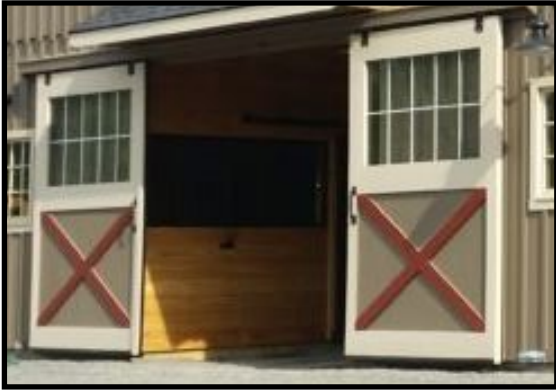
Tempered Glass In Aisle Doors
