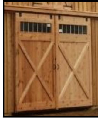
Transom Windows in Aisle Doors
