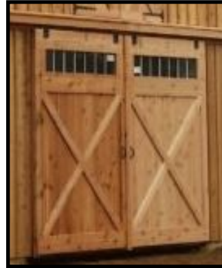
Transom Windows in Aisle Doors
