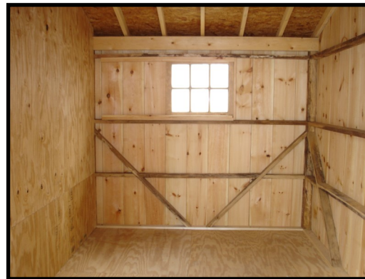
Interior view of tack room
