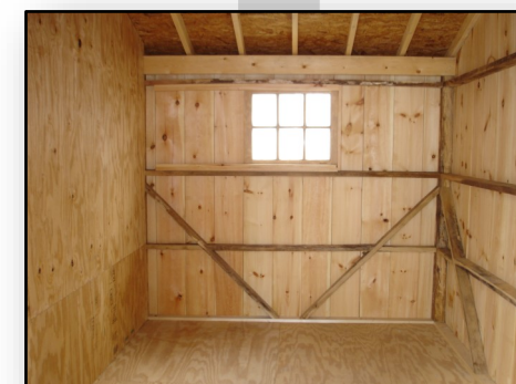
Inside of tack room - One window, full floor, and solid divider wall
