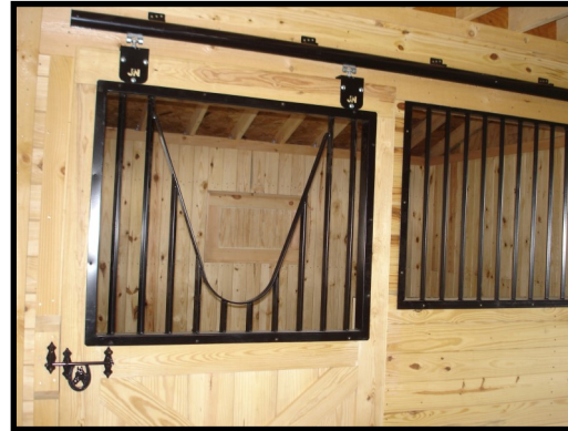
Sliding stall door w/ yoke in door
