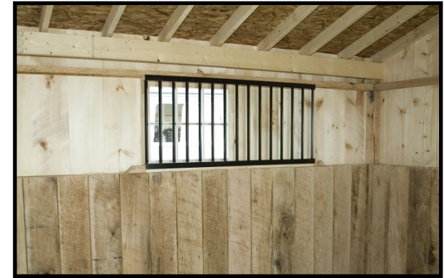
Interior view of 28"x24" standard window w/ metal grill
