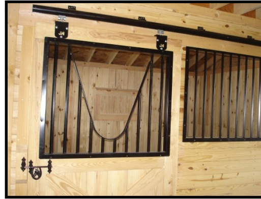
Sliding stall door w/ yoke in door
