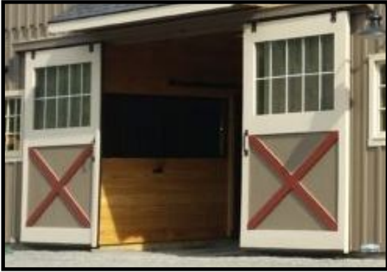
Tempered Glass In Aisle Doors
