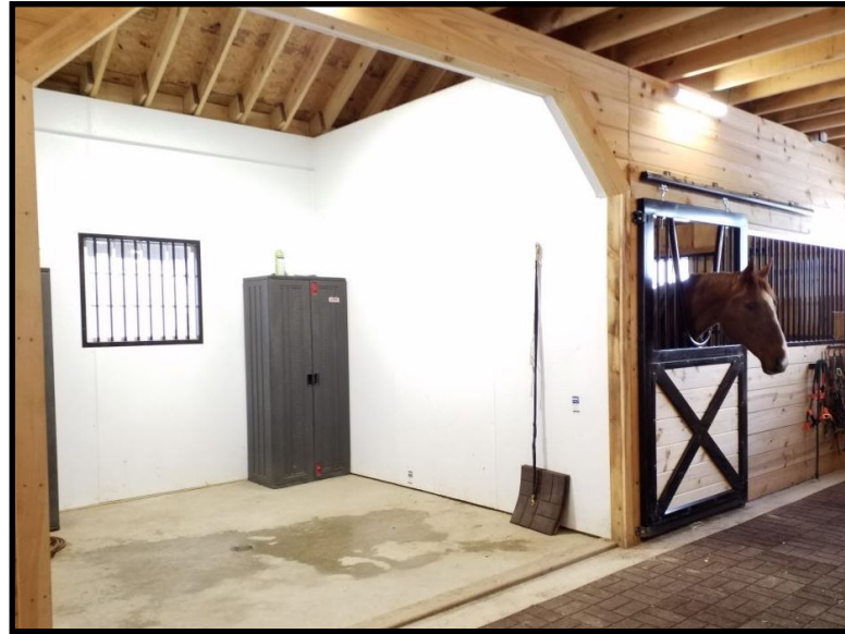
Wash Stall - Moisture Board on Walls - Shown With Window
