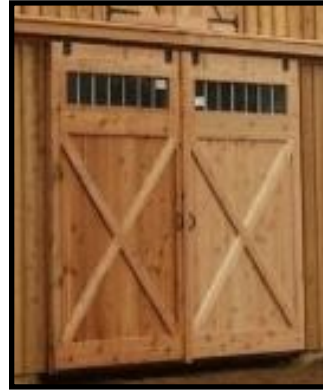
Transom Windows in Aisle Doors
