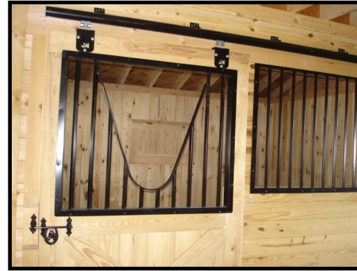
Sliding stall door w/ yoke in door
