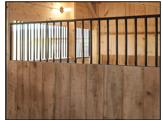
ABOVE: 4' wall with 2' metal grill BELOW: Solid divider wall
