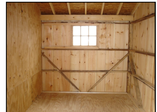
Inside of tack room - One window, full floor, and solid divider wall
