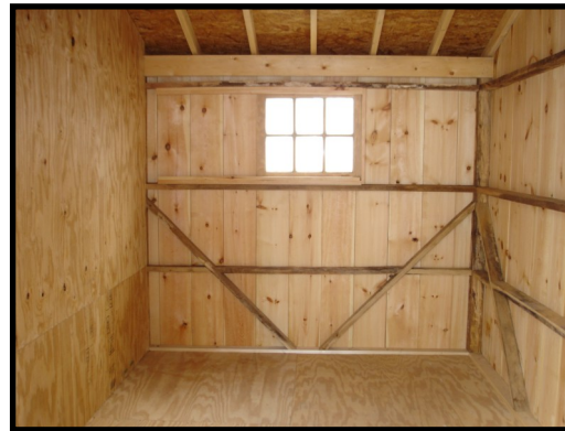
Interior view of tack room
