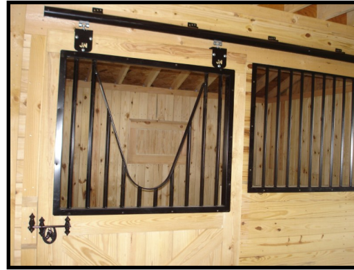
Sliding stall door w/ yoke in door
