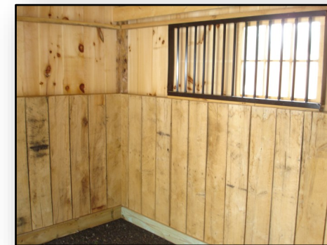
Inside of stall - Kick board and window with metal grill; No floor
