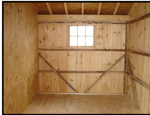
Interior view of tack room
