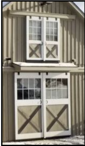
Double Sliding Doors Above Center Aisle
