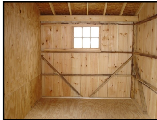
Interior view of tack room
